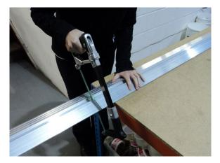
Cut the end aluminium sections to size / shape and cut the two bottom rubber seals and the top cap to the required size.
