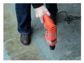
Remove the Threshold Seal and using a 6mm masonry drill bit, drill holes in to the floor where you have marked the ground. (Drill holes are spaced approximately every 200mm and 50mm from each end).
